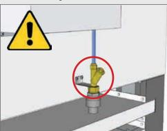
This appliance must be installed with a proper backflow protection system by an authorized personnel
